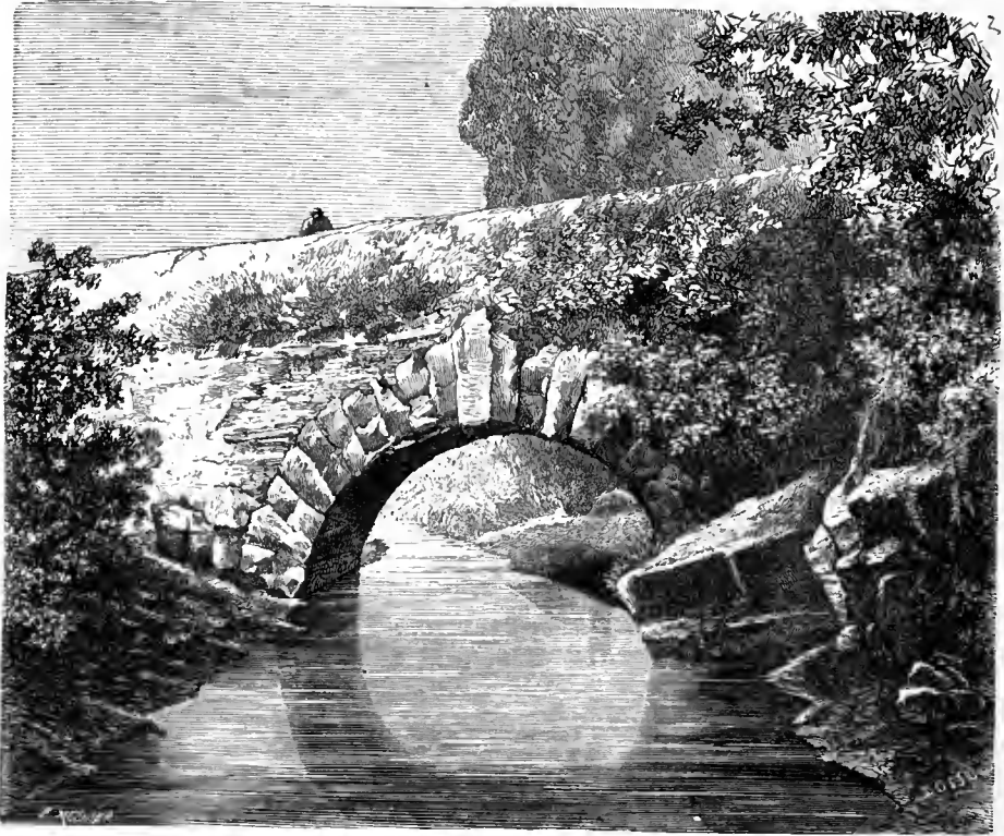
Roman Bridge over the Ostian Road.
